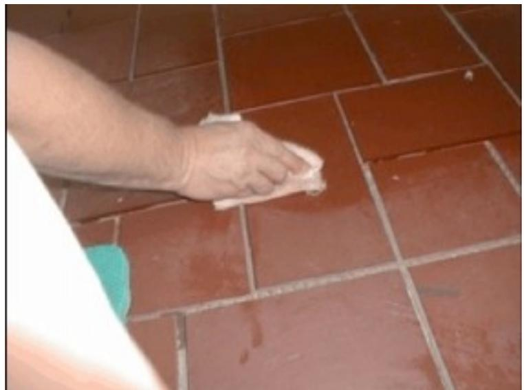
The grout-release agent is easy to work with and dries pretty quickly. You can almost always grout within an hour or two of applying it. Remember, if your ceramic tile has a glazed or shiny surface, there's **NO NEED** to apply a grout-release agent.
