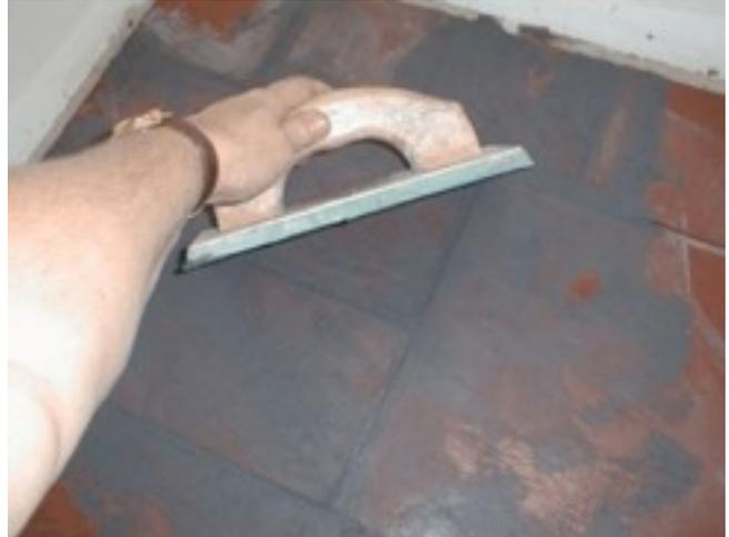
You want the top of the grout at each joint to be flush with the top of the slate or tile on either side of the joint. This will not always be easy as some slate can be thicker than others. You'll see how the rubber float controls this fairly well as you glide it across the slate. Note in the photo, how almost all of the excess grout has been removed from the slate.
