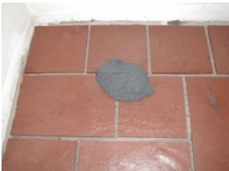
In this photo, you can see I scooped out a glob of grout from the bucket. A 4-inch drywall taping knife is a great tool to use for this purpose. The grout you see in this photo is just about enough to fill the grout lines that are visible in the photo. You only want to apply as much grout as you can spread in an area about 2 feet by 2 feet square. You can always scoop more grout from the bucket, so there's no need to make a huge pile in one spot and move it around.
