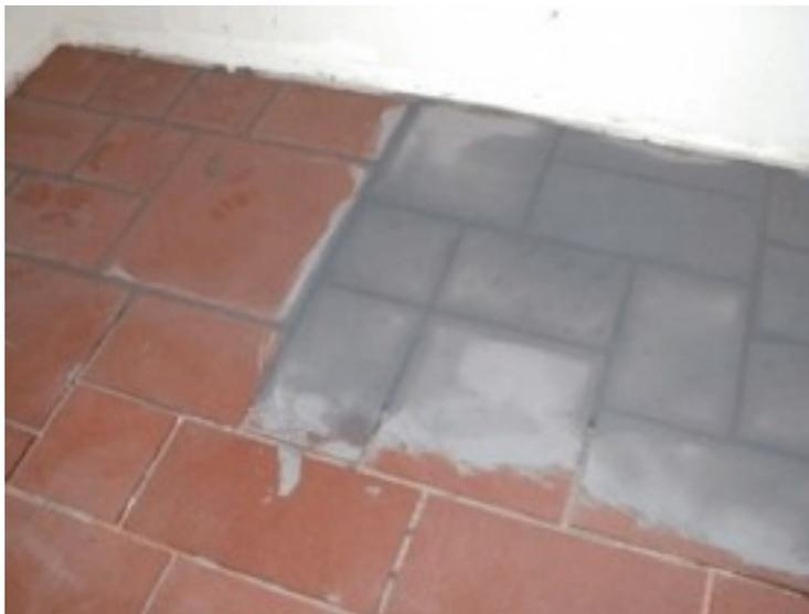
One danger area is putting too much grout onto the slate or tile at once. In other words, filling a large area of the slate without cleaning off the residue from the face of the slate. There's no magic number here. It depends on the humidity of the air, the temperature in the room and how quickly your grout is setting up or getting hard.
