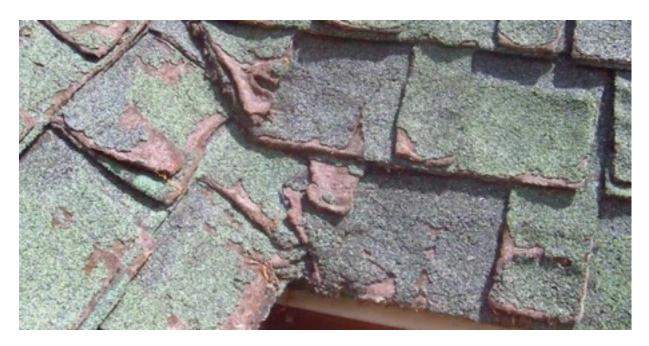
My house roof has a steep 12 / 12-pitch roof and gravity finally won the battle as the asphalt cement used to bond the lower layer to the upper layer of some of the shingles lost its adhesive power.
